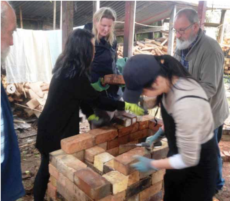
Peter Lange's Diploma students building a small gas-fired soda kiln - it's not a firing module per se, but you can't keep a good kiln-builder down... or a keen bunch of Dipsters, who jumped on the idea (Photo: Thomas Blackstock)
